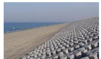
**Sea walls:** Vertical or sloping, shore-parallel structures designed to address erosion and flooding hazards. Vertical designs cause more reflection of incoming wave energy and may lead to scouring of the beach in front of the wall, while sloping designs are more capable of disseminating the incoming energy.
