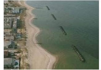
**Groynes:** hard structures perpendicular to the coast to trap longshore sediment transport to address erosion. The downsides are the possibility on sediment starvation downstream, and the formation of rip currents adjacent to the groynes that can lead to sediment loss and dangerous situations for swimmers.
