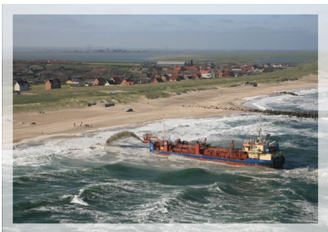
Beach nourishment with Trailing Suction Hopper Dredger (Photo: Rohde Nielsen).
