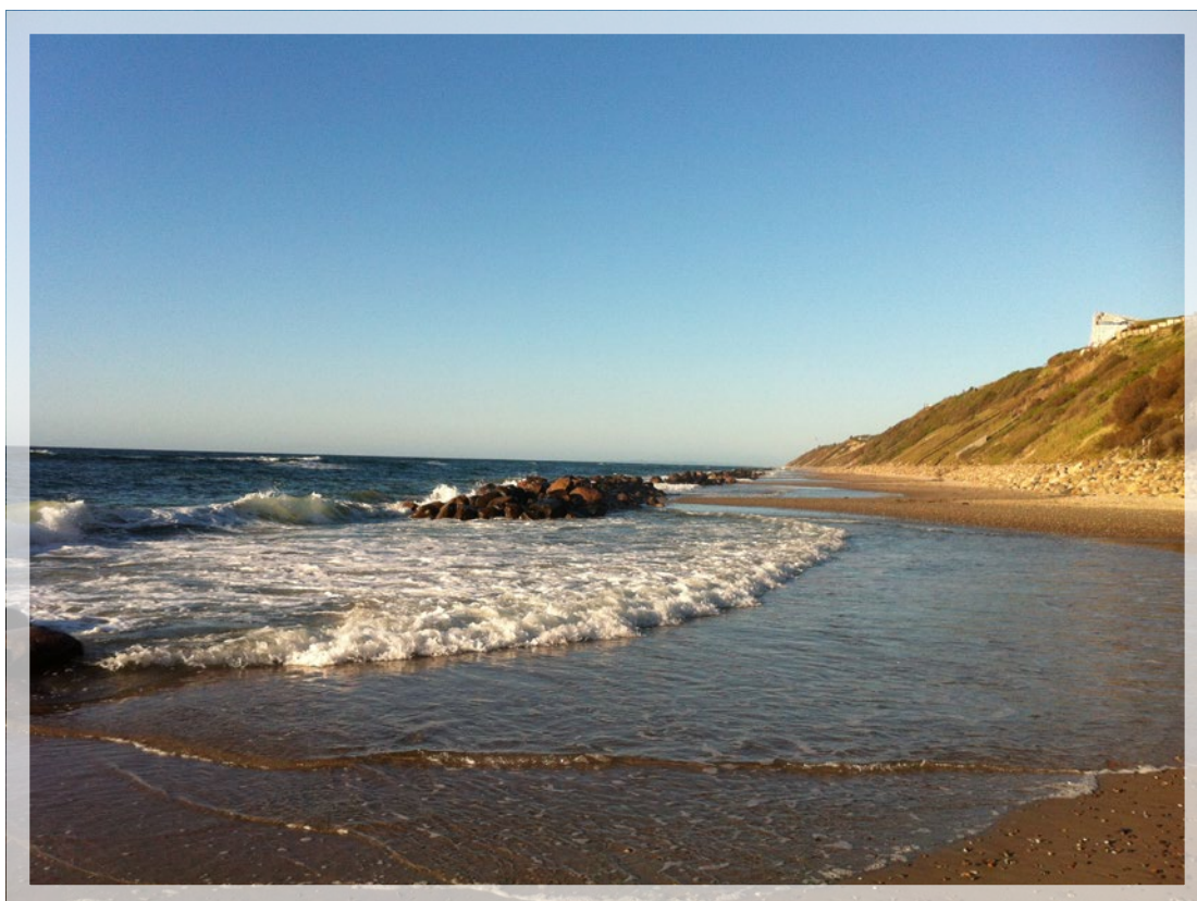
Fig. 2.2. Breakwater structures in Denmark.
