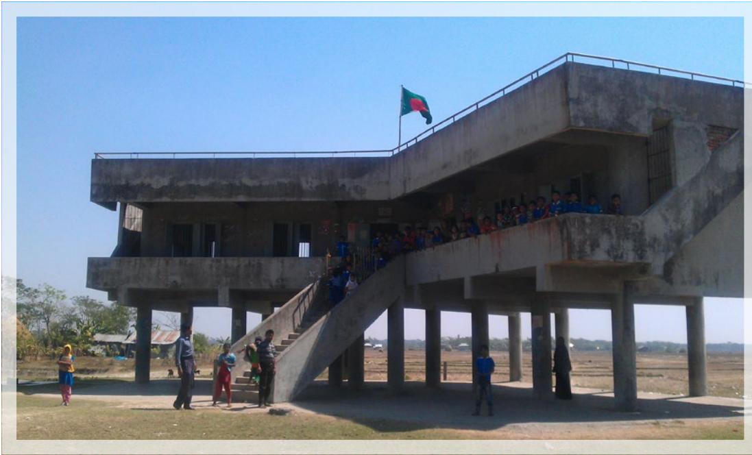
Fig. 12.1. Flood shelter structure (Photo: Helena Wright 2013, CC BY 2.0).
